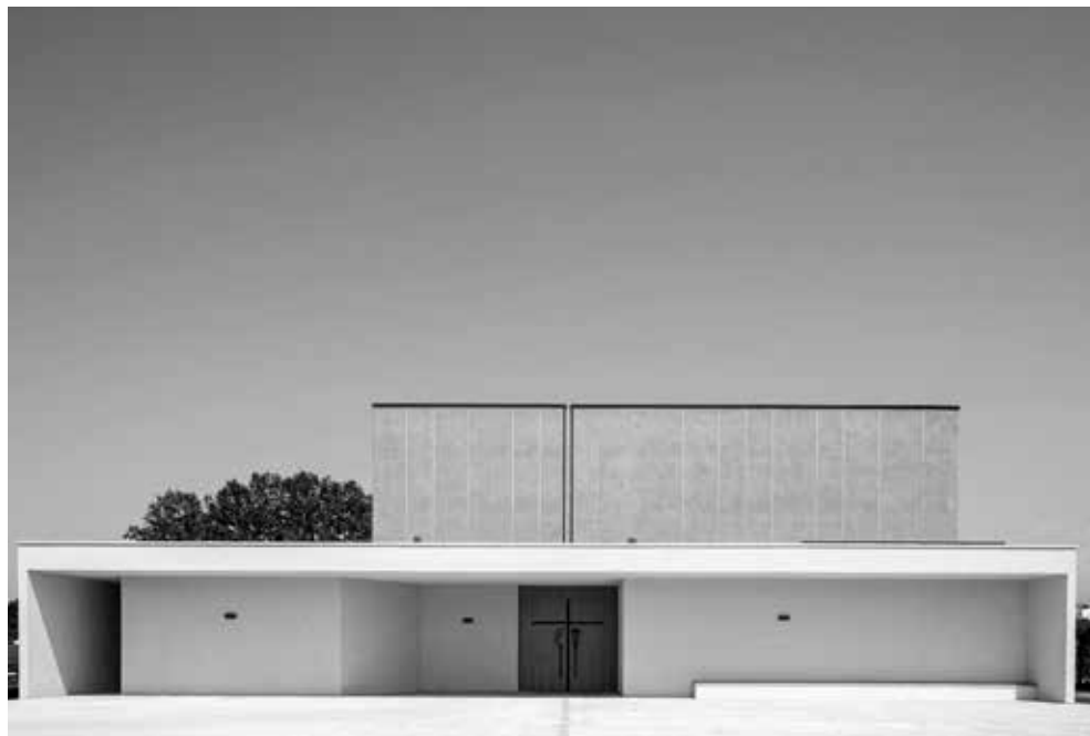
Ill. 3. Church of Resurrection of the Lord in Viareggio, Italy, proj. Studio TAMassociati, phot. Andrea Avezzù, courtesy of Studio TAMassociati.
