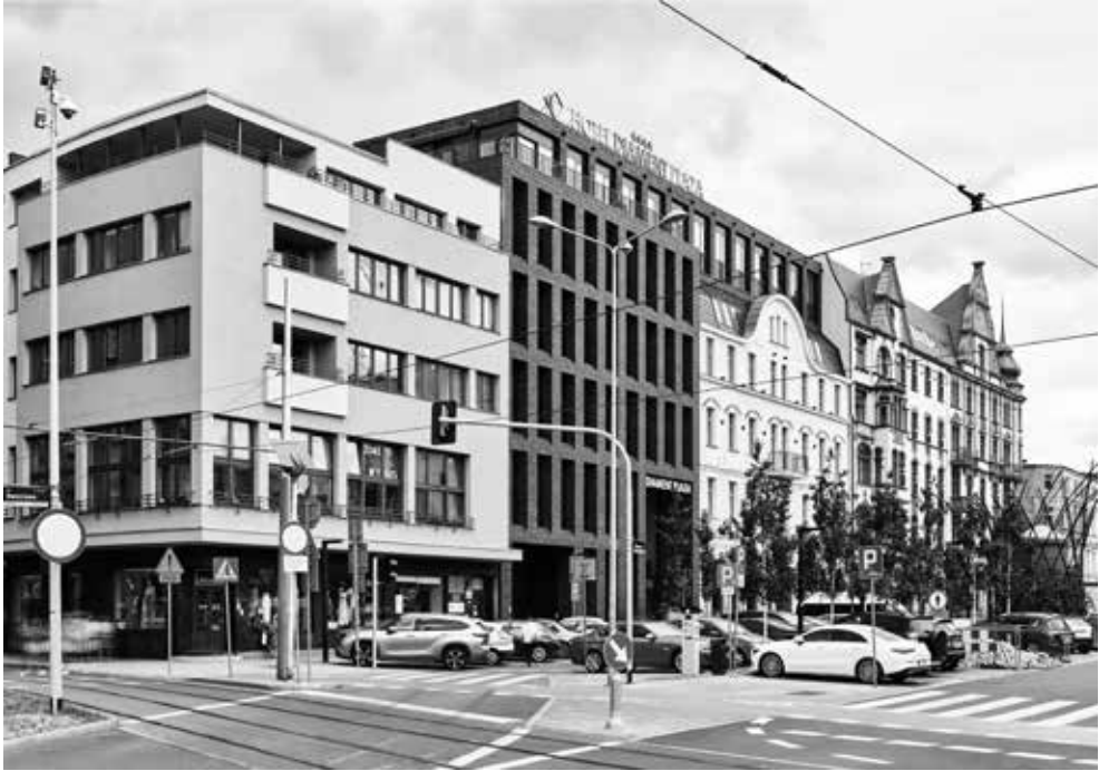
Ill. 3. Diamant Hotel Plaza in Katowice, designed by Konior Studio, realization: 2021. Photography by: Jakub Certowicz.
