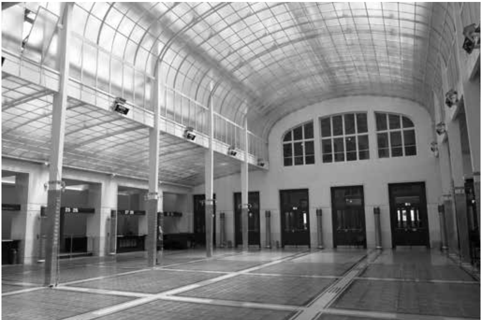
Ill. 4. The main banking hall in the Postsparkasse building with a skylight and a glass floor (source: photo by author, 2015).
