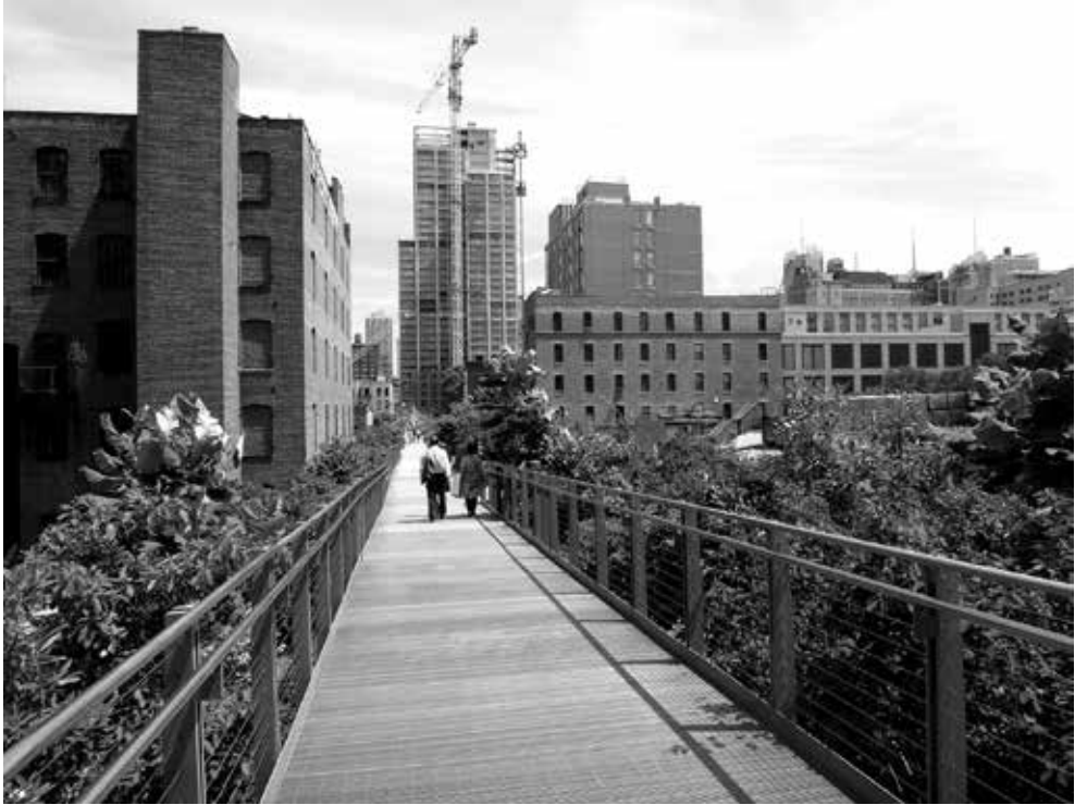
Ill. 4. View of the High Line flyover in New York City, buildings under construction are visible in the background (photo: author).
