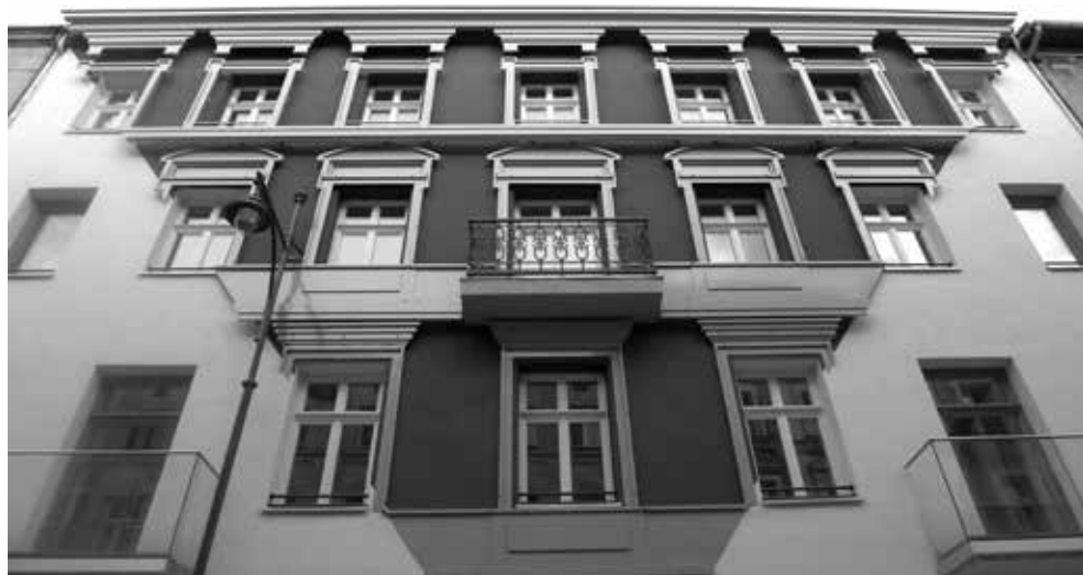
Ill. 2. Building at 15 Włókiennicza Street, photo by Anna Mielnik.
