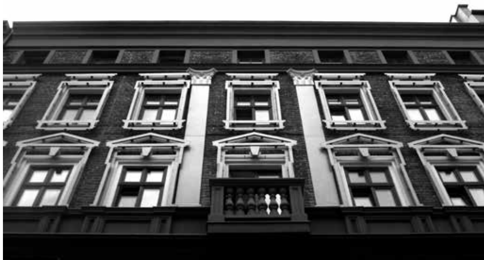
III. 3. Building at 14 Włókiennicza Street, photo by Anna Mielnik.
