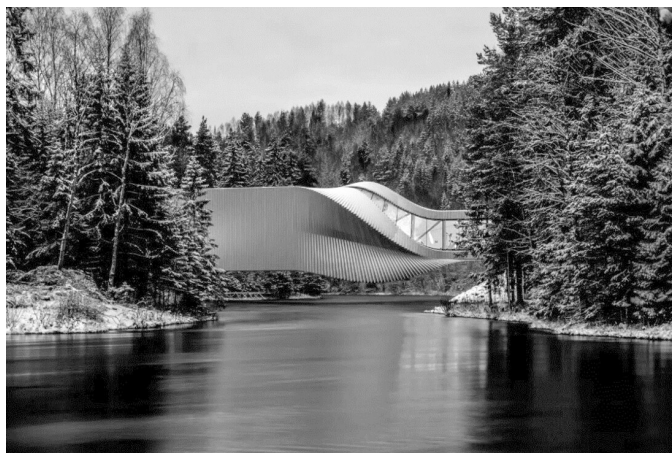
Ill. 6. Kistefos Art Museum – “The Twist”; source: The Twist [in:] BIG – Bjarke Ingels Group, https://big.dk/projects/the-twist-1337 (access: 7.08.2024).
