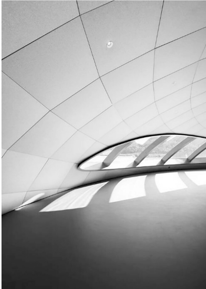
Ill. 11. Salmon Eye – interior: view of acoustic panels, source: S. Utkum Ikiz, Salmon Eye, a spectacular floating pavilion on Hardangerfjord [in:] Parametric Architecture, 3.12.2022, https://parametric-architecture.com/salmon-eye-a-spectacular-floating-pavilion-on-hardangerfjord/ (access: 7.08.2024).
