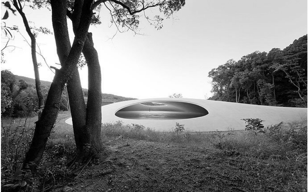
Ill. 7. The building structure of the Art Museum on the Japanese island of Teshima, architect: Ryue Nishizawa, SANAA, Rei Naito, source: ArchDaily, 19.07.2011, https://www.archdaily.com/151535/teshima-art-museum/1311025649-17teshima-museum-rna-1291.jpeg?next_project=no (access: 15.07.2024).
