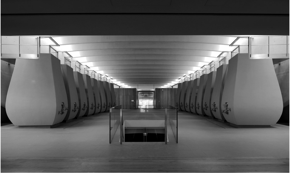
III. 14. Château Cheval Blanc, view of concrete vats, source: Chateau Cheval Blanc Winer / Christian de Portzamparc [in:] ArchDaily, 9.12.2013, https://www.archdaily.com/455019/chateau-cheval-blanc-winer-agences-elizabeth-christian-de-portzamparc (access: 10.06.2024).
