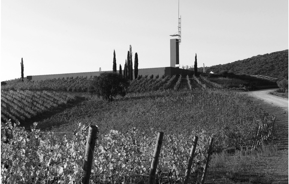
Ill. 9. Rocca di Frassinello, perspective view, source: Rocca di Frassinello Winery [in:] archilovers, https://www.archilovers.com/projects/107957/rocca-di-frassinello-winery-gallery?2266260 (access: 10.06.2024).
