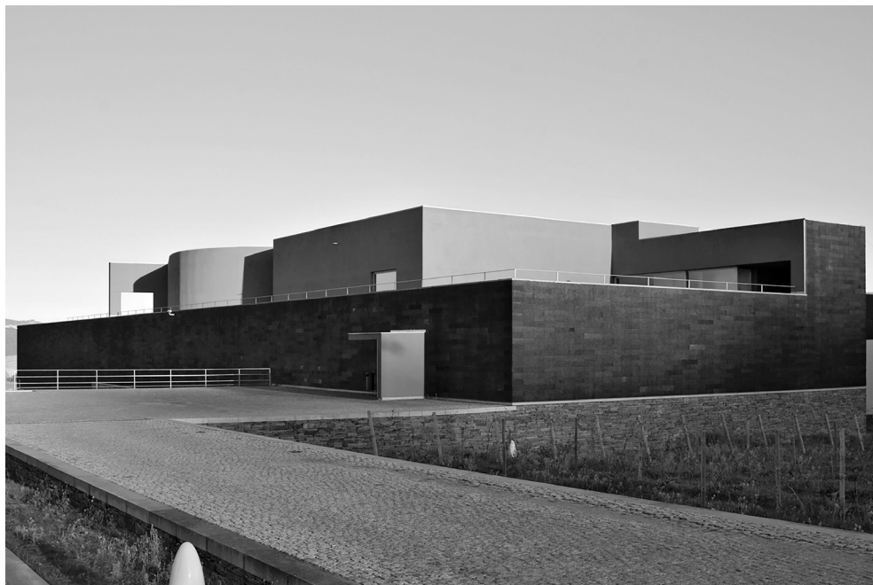
III. 7. Quinta do Portal, perspective view, source: Siza A., Quinta do Portal Winery [in:] archiweb, https://www.archiweb.cz/en/b/vinarstvi-quinta-do-portal-adeqa-quinta-do-portal (access: 10.06.2024).
