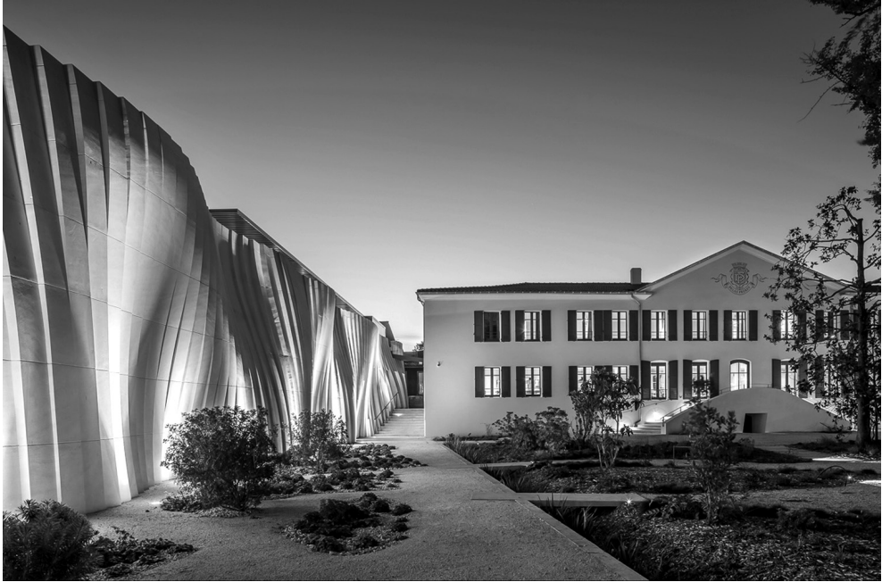
III. 16. Délas Frères, view of the stone wall and historic manor house, source: P. Pintos, Delas Frères Winery / Carl Fredrik Svenstedt Architect [in:] ArchDaily, 13.02.2020, https://www.archdaily.com/933696/delas-freres-winery-carl-fredrik-svenstedt-architecte (access: 10.06.2024).
