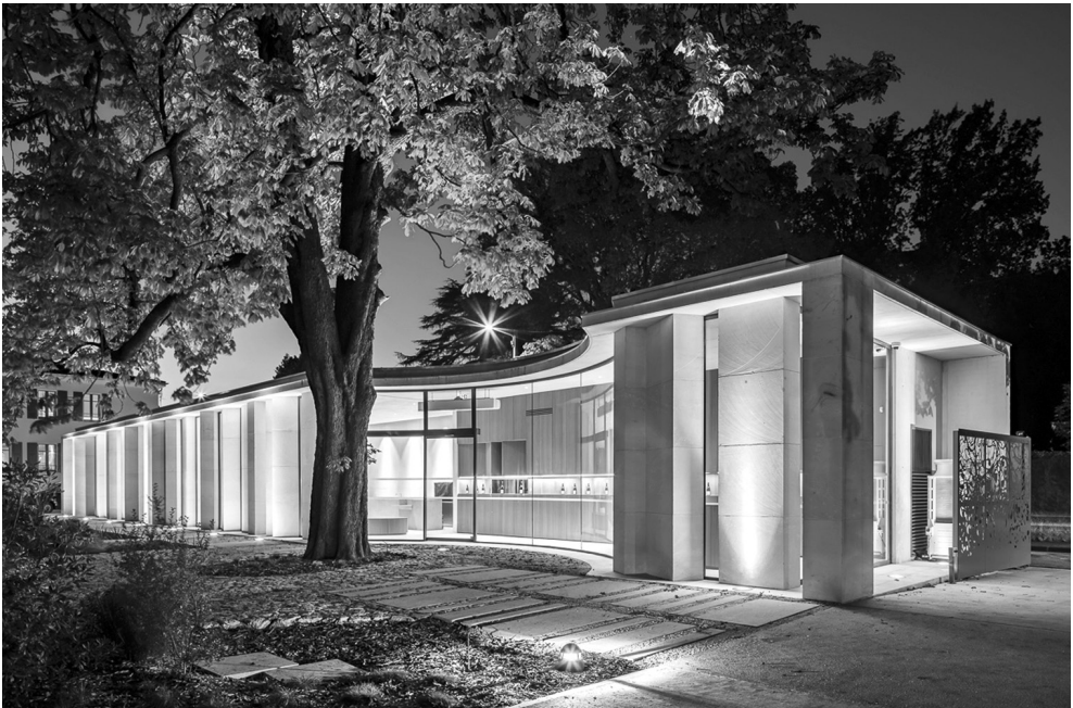
III. 15. Délas Frères, view of the store, source: Chateau Cheval Blanc Winer / Christian de Portzamparc [in:] ArchDaily, 9.12.2013, https://www.archdaily.com/455019/chateau-cheval-blanc-winer-agences-elizabeth-christian-de-portzamparc (access: 10.06.2024).
