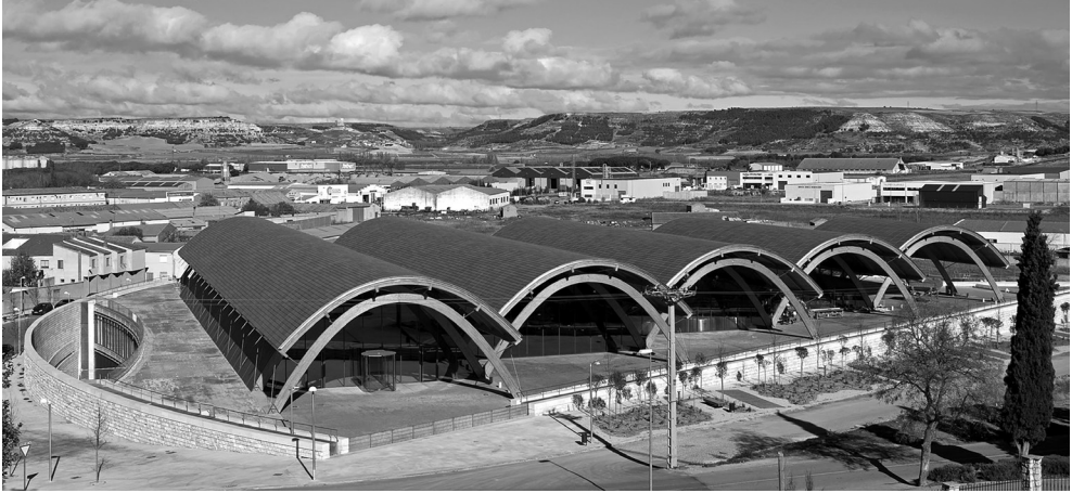
III. 3. Bodegas Protos, front elevation, source: Protos Winery / Richard Rogers + Alonso, Balaguer y Arquitectos Asociados [in:] ArchDaily, 29.04.2014, https://www.archdaily.com/500502/bodegas-protos-richard-rogers-alonso-y-balaguer (access: 10.06.2024).
