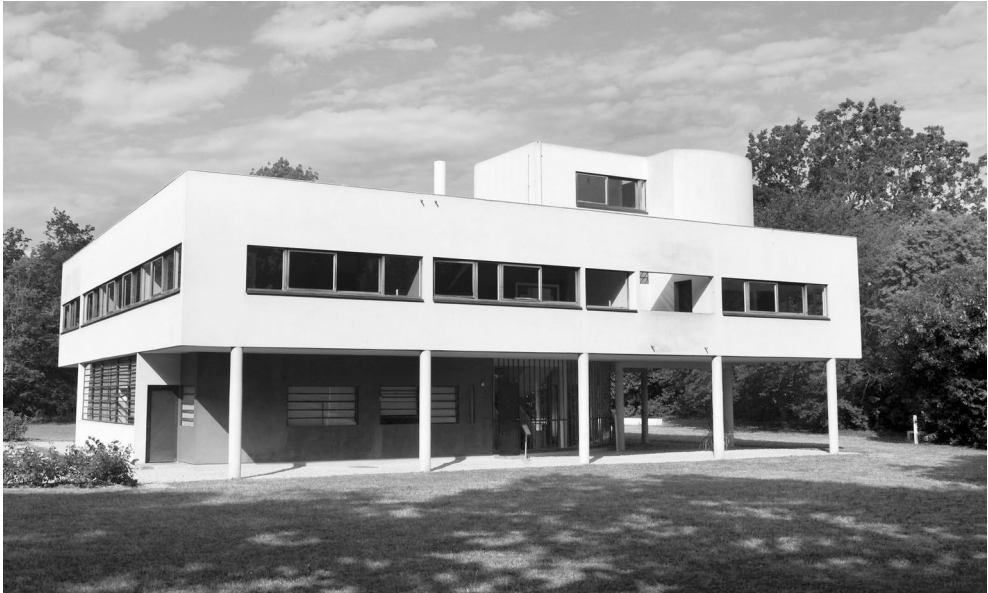
Ill. 1. Villa Savoye , Poissy, France, 1928–1931, design: Le Corbusier. General view – an example of the implementation of the five principles of modern architecture according to Le Corbusier, photo by Tomasz Kozłowski.
