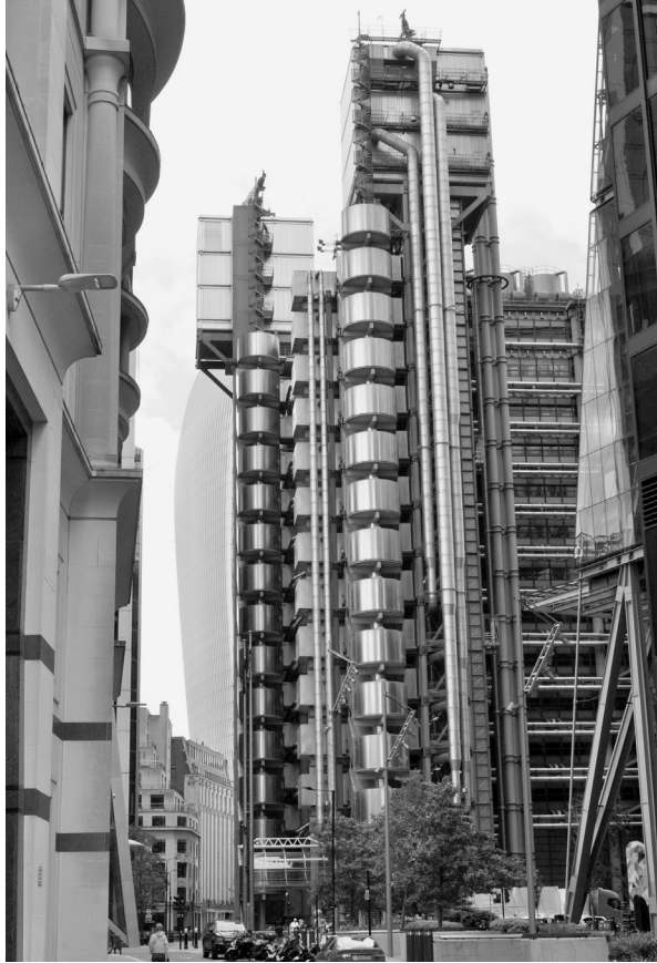
Ill. 2. Lloyd's Building , London, United Kingdom, 1978–1986, design: Richard Rogers & Partners. General view – an example of high-tech aesthetics, photo by Marek Początko.
