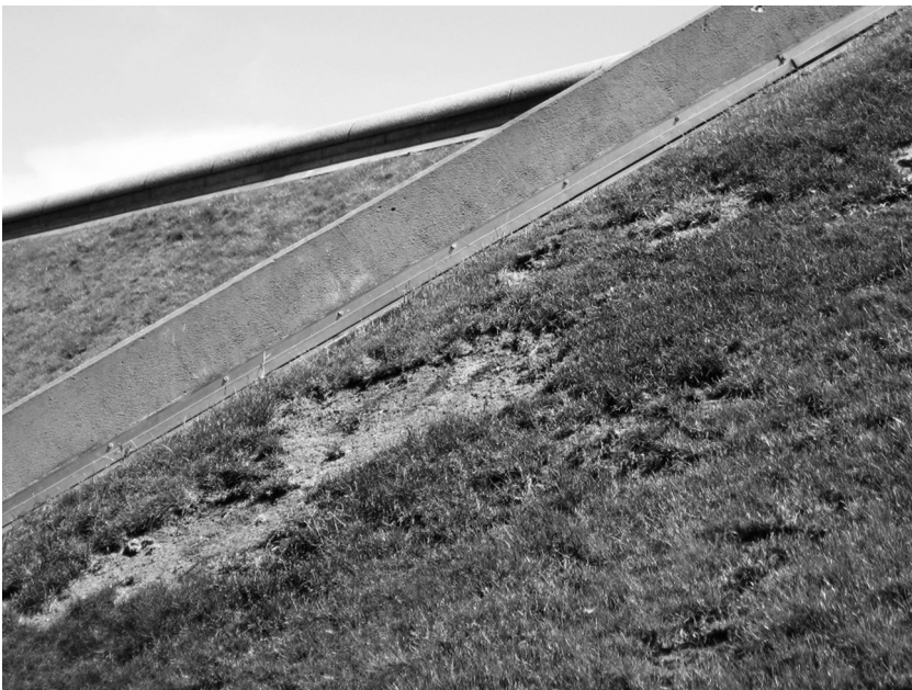
Ill. 5. Palais Omnisports de Paris-Bercy (now Accor Arena), Paris, France. A fragment of the wall shows the problems with maintaining an impeccably trimmed lawn on the steep wall of the building, photo by R. Mikielewicz, 2010.
