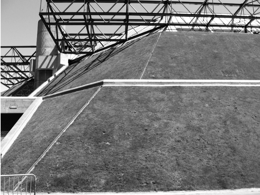
Ill. 4. Palais Omnisports de Paris-Bercy (now Accor Arena, proj. architectural office Andrault-Parat, J. Prouvé, A. Guvan, 1984), Paris, France. A fragment of the façade with visible imperfections in the immaculate green lawn on the unusually steep wall, photo by R. Mikielewicz, 2010.
