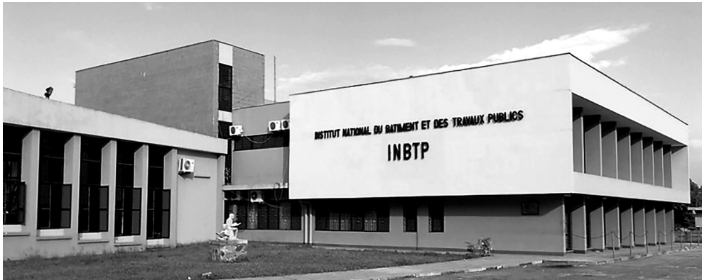
Ill. 4. View of the Administration block of the INBTP Complex in Kinshasa by Eugene Palumbo, source: Victor Bay, 2024.
