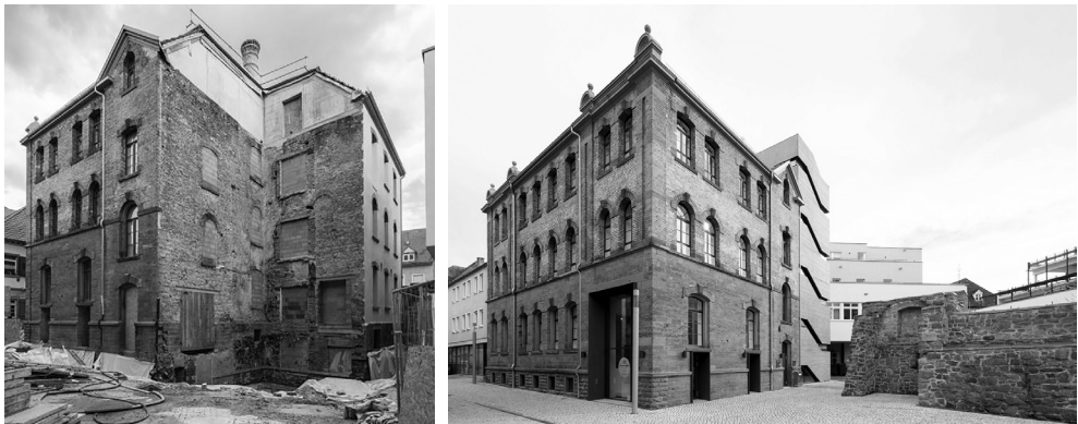
III. 9. Reconstruction of the Tonofenfabrik brick factory into a museum (Lahr, Germany). The existing part of the building has been renovated, supplemented by a new stair tower made of red concrete, source: M.F. González, Museum Tonofenfabrik Lahr / Heneghan Peng Architects [in:] ArchDaily, 3.09.2018, https://www.archdaily.com/901070/museum-tonofenfabrik-lahr-heneghan-peng-architects (access: 1.10.2024).
