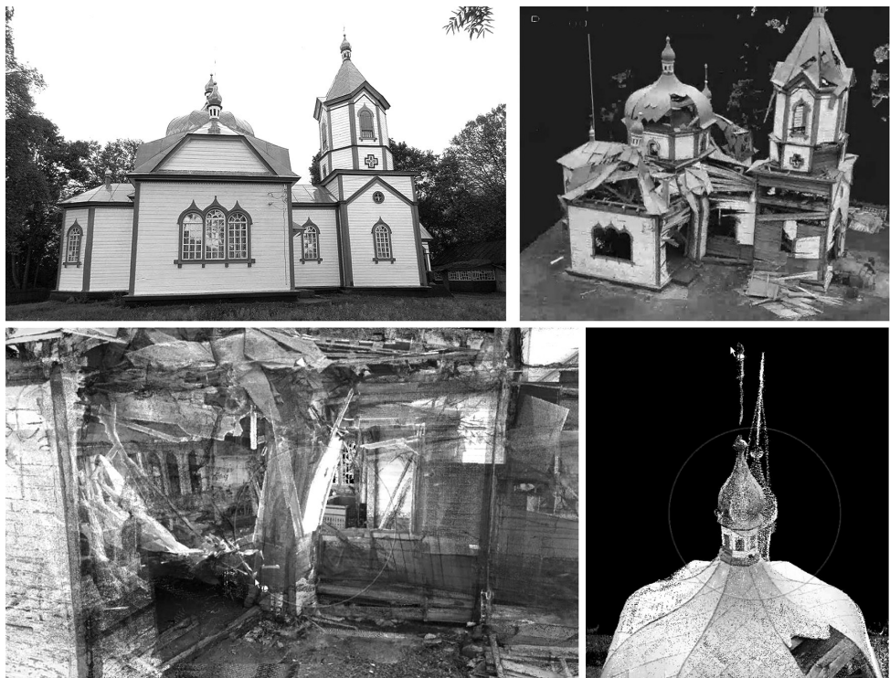
Ill. 5. Church of the Nativity of the Holy Mother of God, Viazivka village, Zhytomyr region: general view, photogrammetry (May 2023), Laser scanning (October 2023). Vasyl Rozhko, source: V. Rozhko et al., Heritage monitoring for restoration... , op. cit., p. 17.
