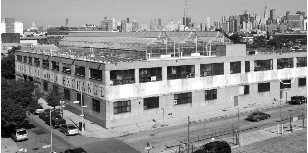
III. 3. Gotham Greens rooftop farm in Greenpoint, source: 810 Humboldt Street [in:] Greenpoint Manufacturing and Design Center, https://gmdconline.org/gmdc_buildings/810-humboldt-street (access: 30.06.2024).
