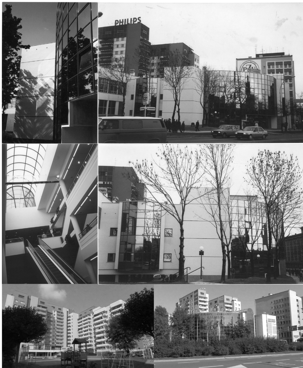
III. 4. BI Unit Rzeszów Centre residential and commercial complex – “Ameryka” Shopping Centre at 40 Józefa Piłsudskiego Avenue and residential buildings at 7 Stanisława Jabłońskiego Street, main designer and author: arch. Mieczysław Gała, co-author collaboration arch. Witold Sztorec; photos: Mieczysław Gała, Monika Gała-Walczowska.
