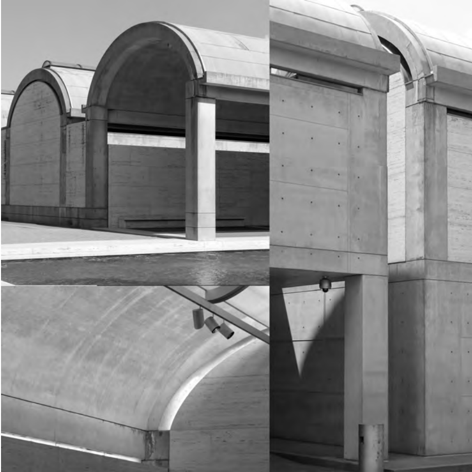
Ill. 4. Window slits below the vaults of Kimbell Art Museum, Fort Worth, from the outside and inside, photo by M. Pieczara, 2007.
