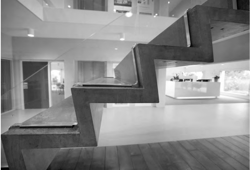
Ill. 7. Slim and light hybrid stairs by ABT, made of UHPC concrete and Si-X architectural glass, source: Ultra-slim hybrid staircase [in:] ABT Consulting engineers, https://www.abt.eu/en/expertise/innovations/ultra-thin-hybrid-staircase.aspx (access: 30.05.2024).
