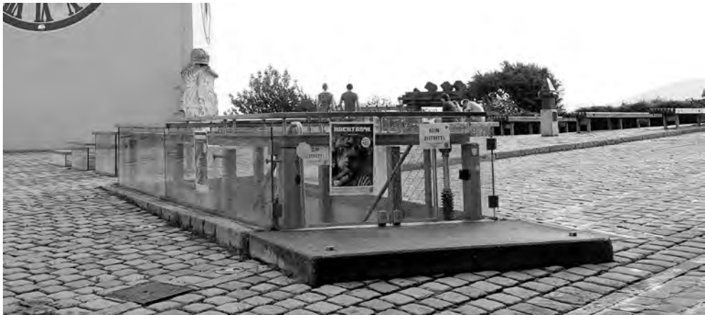
Ill. 2. Stairs with a hydraulically controlled roof, Schloßbergsteig castle, Graz, Austria, 2018, photo by P. Opalka.
