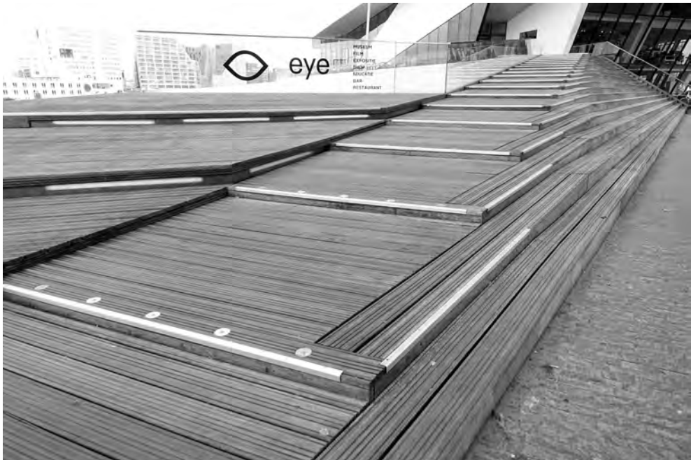
Ill. 3. Combination of three types of external stairs, EYE Museum, Amsterdam, 2017, photo by P. Opalka.
