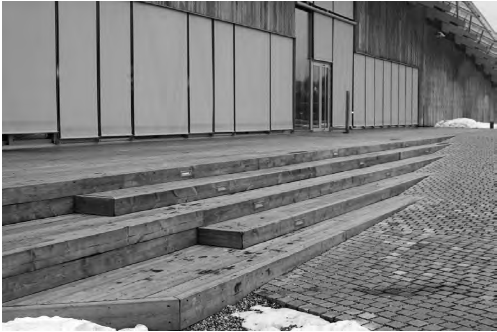
Ill. 4. Wooden external stairs leading into the auditorium and connecting with the ramp, Astrup Fearnley Museet, Oslo, design: architect R. Piano, 2014, photo by P. Opalka.
