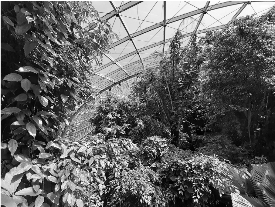
Ill. 1. Covering in the rainforest pavilion – Tiergarten Schönbrunn, Vienna, photo: M. Gyurkovich.
