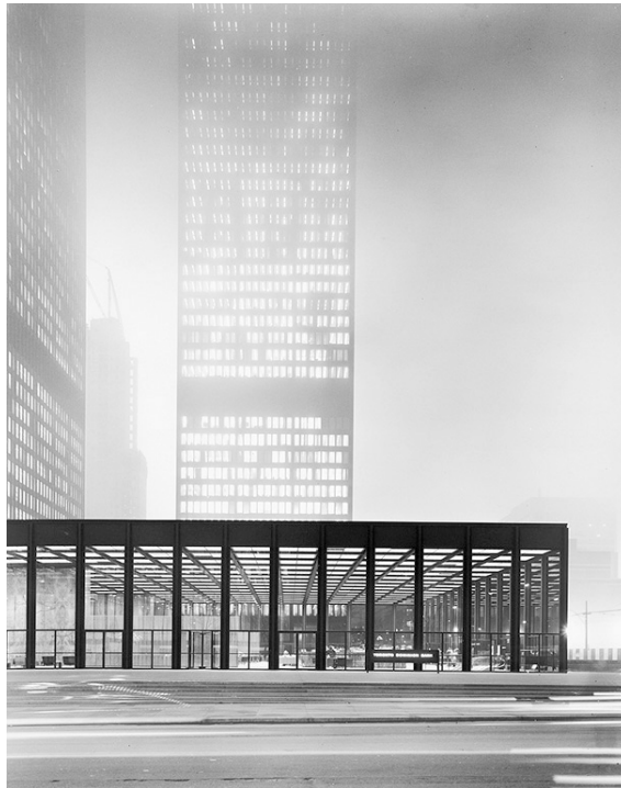
III. 4. L. Mies van der Rohe, Dominion Center Toronto, Canada (1963–1969), photo B. Korab 1973, Library of Congress, https://www.loc.gov/resource/ppem.00695/ (access: 15.10.2024).
