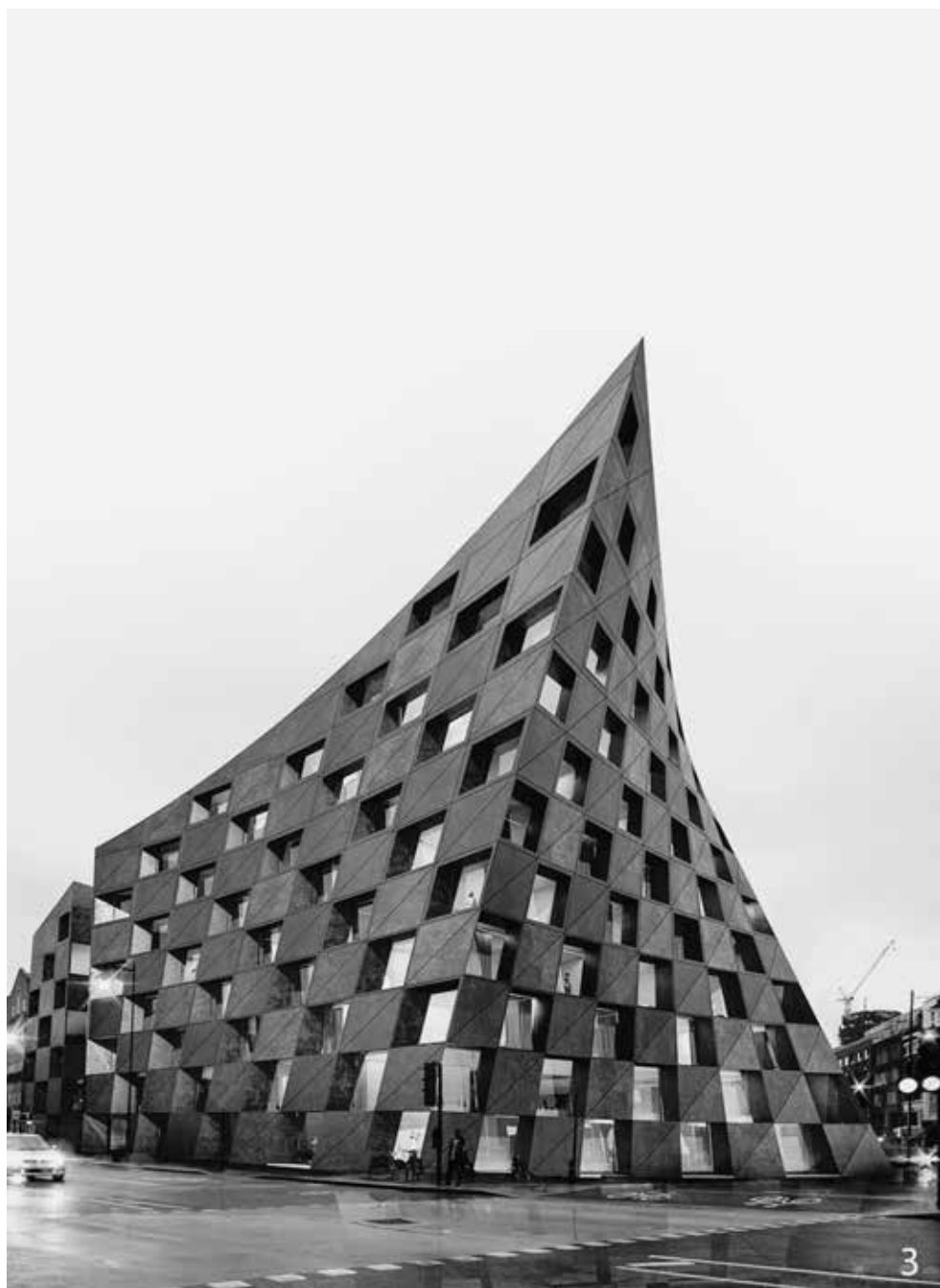
III. 3. AQS0 Arquitectos, Shoreditch Hotel , London, 2017 http://www.archdaily.com/ (access: 2.5.2020)
