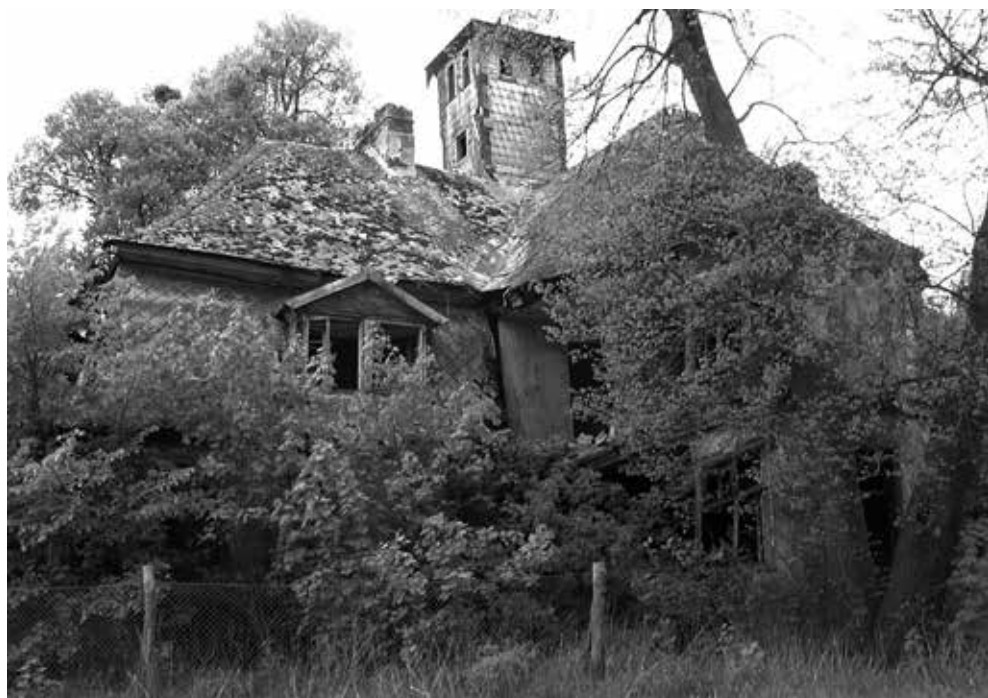
III. 2. Manor house in Łopuchowo – 2005, photo: P. Zierke
