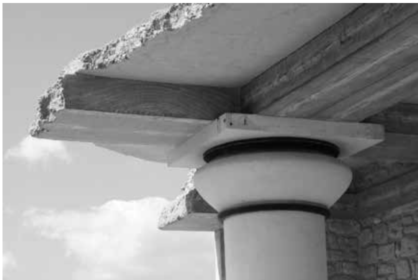
III. 3. Concrete entablature and column head detail, Knossos Palace, Crete, author's photo, 2009
