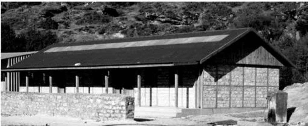
Ill. 3. A school building in Khumjung designed by Shigeru Ban Architects. Source: own materials
