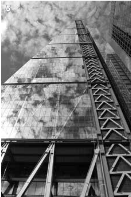
Ill. 5. Structural elements in facade of the Leadenhall Building, photo by author
