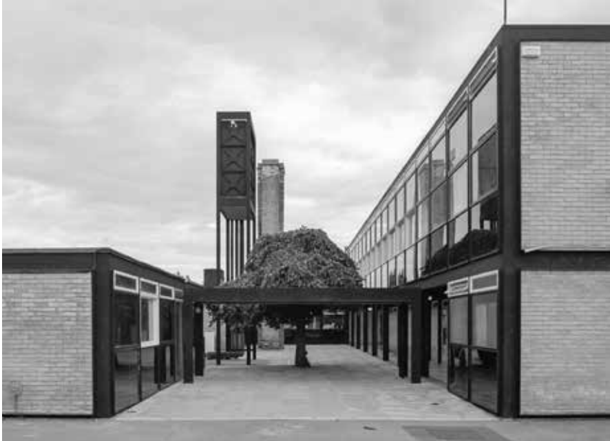
III. 3. Alison Smithson and Peter Smithson, Secondary School in Hunstanton (water tank and chimney in the center of the photo), 1949–1954; photo by Xavier de Jauréguiberry
