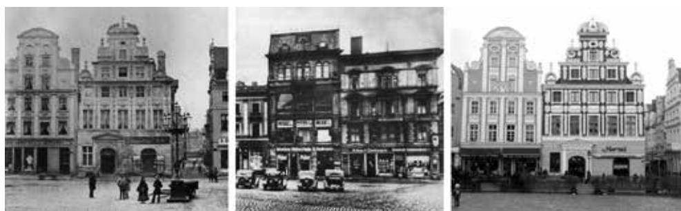
III. 3. Kołobrzeg. Architecture on the same plots at the beginning of the 20th century, in the 1970s and nowadays: after demolition of the old town houses, a commercial house was built, whose reinforced concrete structure was adopted for the function of a production plant, transformed into a shopping center, [in:] https://miastokolobrzeg.pl (online 14.08.2020, fragments), author's photography
