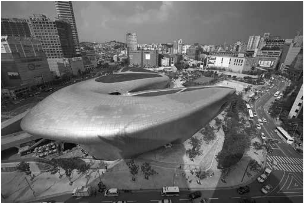
III. 2. Zaha Hadid, Dongdaemun Design Park, Seoul, 2009–2014. A building detached from context, ignoring the tradition and history of the place, similar to other works of Hadid (e.g. Opera House in Guangdong) but visually attractive. The construction of this world's biggest atypical building devoured the entire area of the municipal park ( https://divisare.com/projects/328000-zaha-hadid-architects-julien-lanoo-dongdaemun-design-plaza#lg=1&slide=3 , access: 31.01.2020.)
