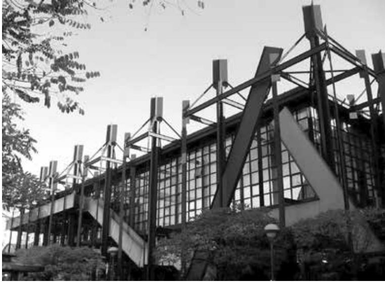
Ill. 3. School of Architecture, Polytechnic of Milan, Viganò, 1970–1985. From Corriere della Sera , 2020 (an interpretation of the image made by O. Longo)
