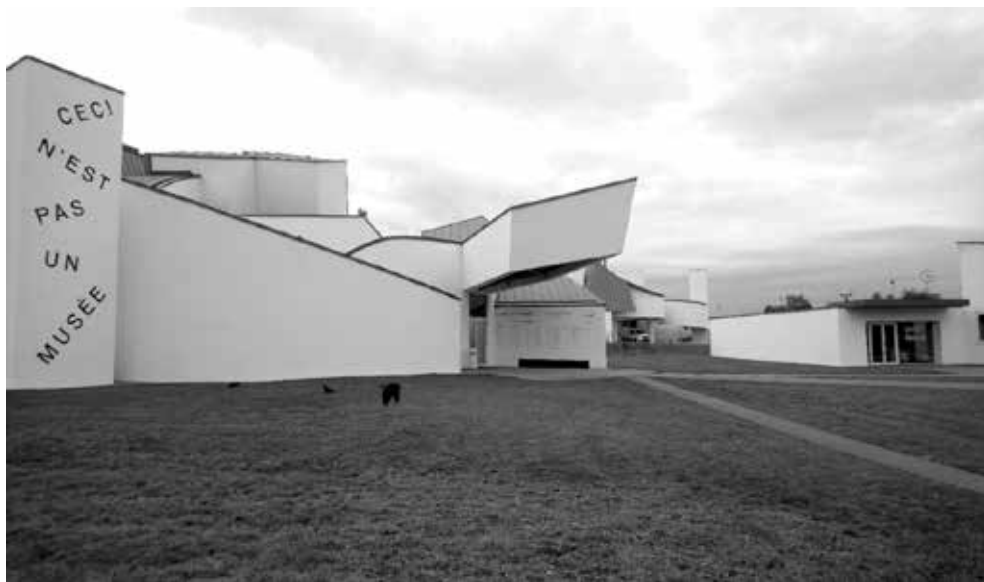
III. 4. Semantic deconstructivism. The acontextual form of a kind of artistic manifesto. The second stage of simulation: the externally perceived form is not a reflection of the internal spatial and functional system, suggesting, however, the existence of such a system, it reflects the non-existent relationships of the constructed copy of the alleged reality with the real one. The simulacrum is a distortion of reality. Vitra Design Museum ; designed by Gerry Partners; photo: G. Nawrot
