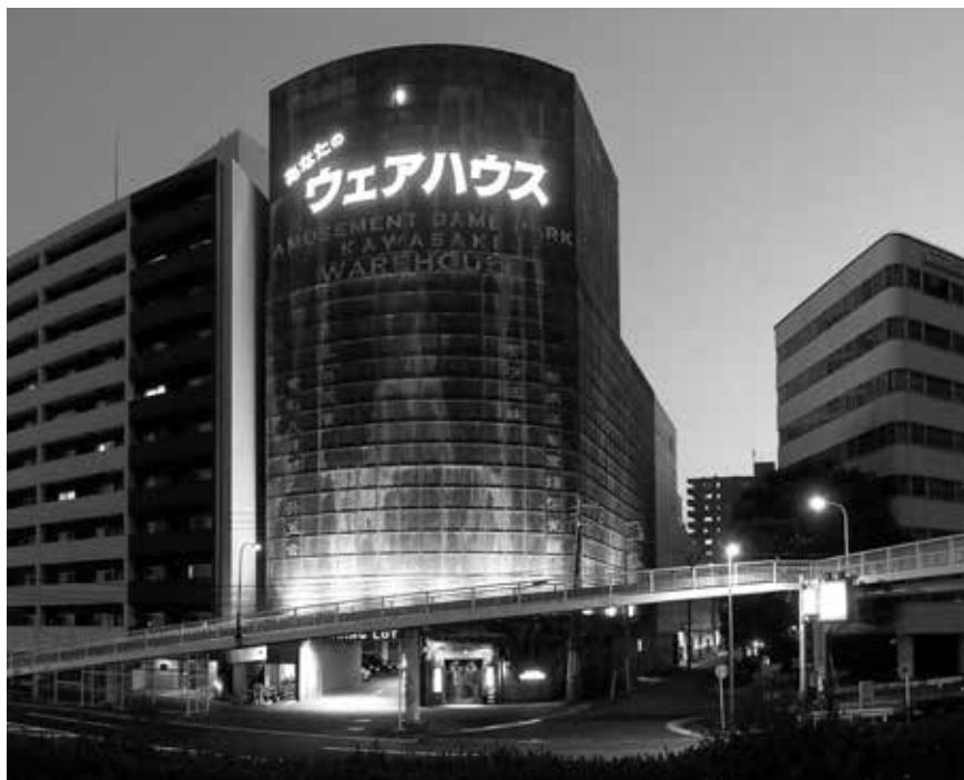
III. 2. Kawasaki Warehouse, (photo: Ken Ohyama)
