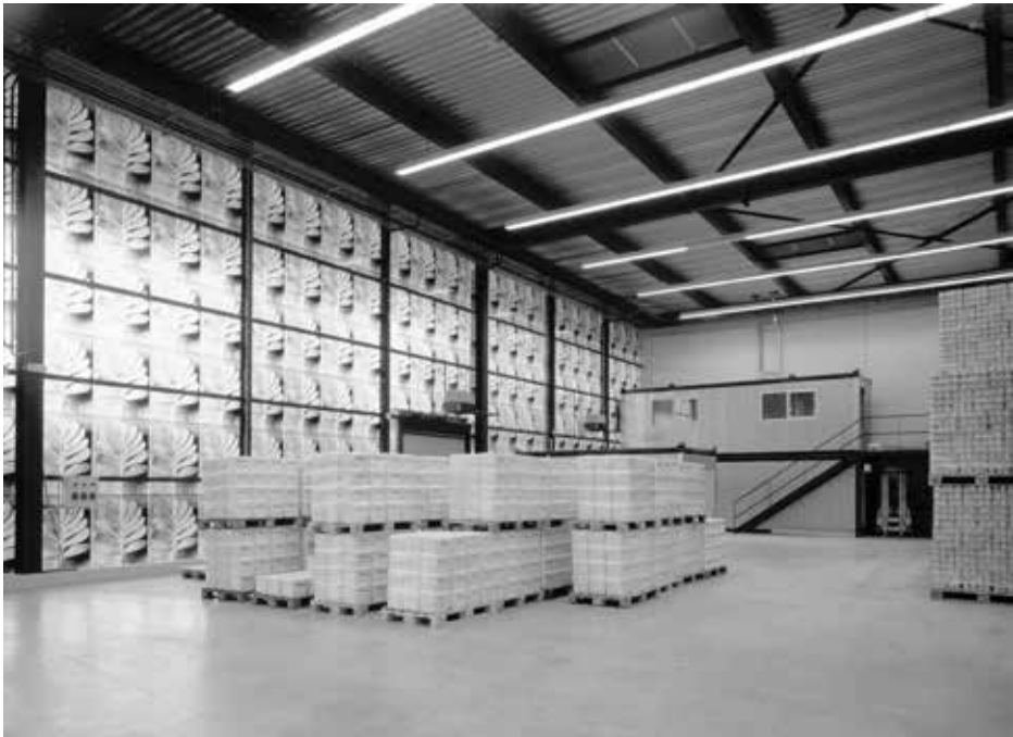
Ill. 2. The interior of the Ricola-Europe SA, Production and Storage Building Mulhouse-Brunstatt, France, Project 1992, realization 1993. Source: Margherita Spiluttini photographer
