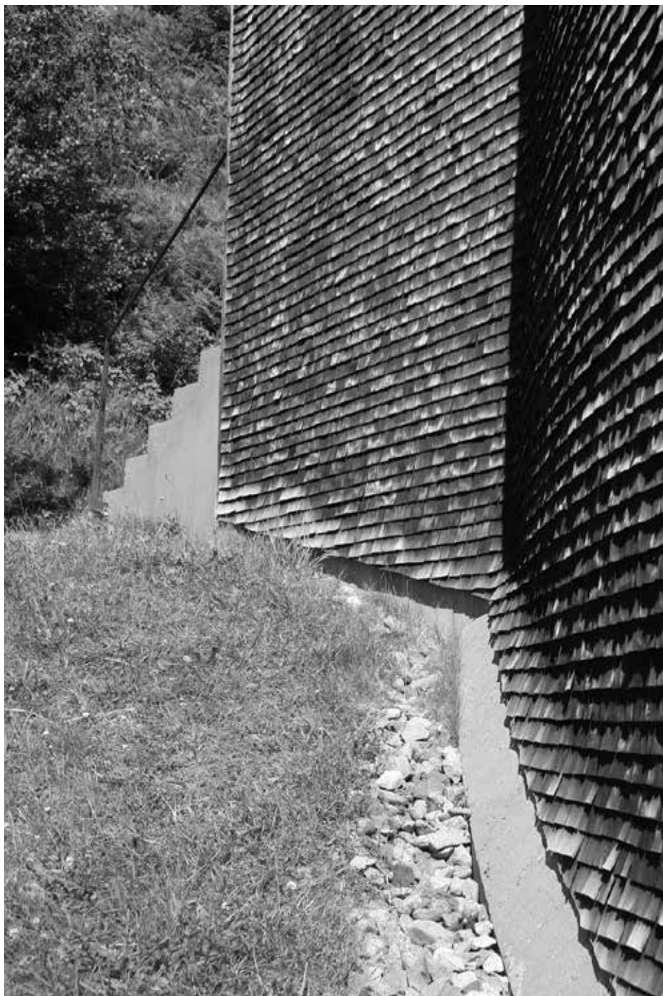
Ill. 12. Sogn Benedetg in Sumvitg chapel by P. Zumthor, detail, author's photo.
