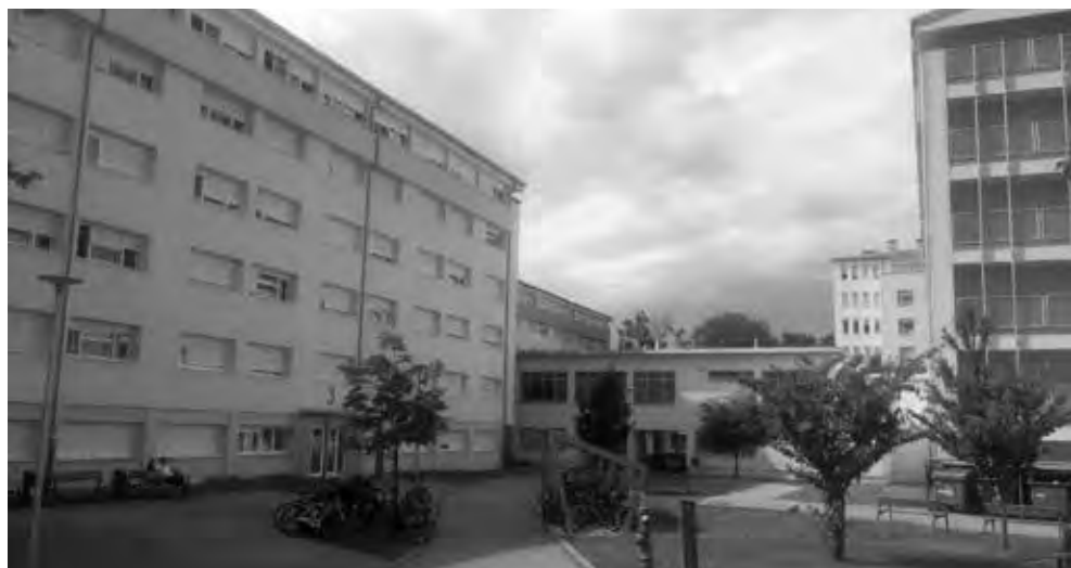
Ill. 3. Students Residence Hall Cvjetno naselje, Author's Archive (photo 2022).
