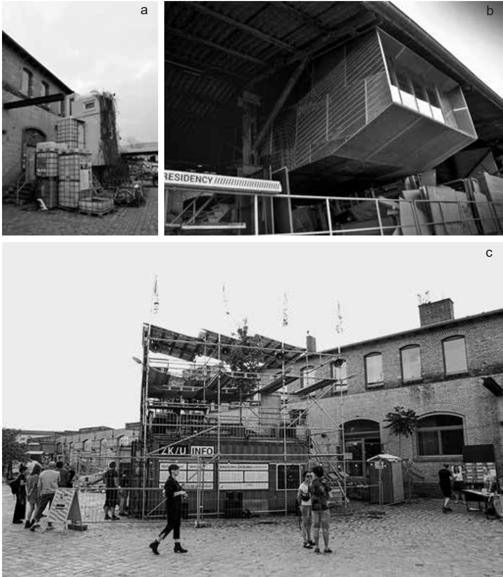
III. 6. Zentrum für Kunst und Urbanistik, Berlin: a) Jan Körbes, Silo Haus, author's photo; b) workshop hall – “parasitic architecture” from school boards suspended to the roof of the old platform, author's photo; c) Municipal Stage, source: https://www.zku-berlin.org/projects/construction-explained-urban-stage/ (access: 10.05.2022).
