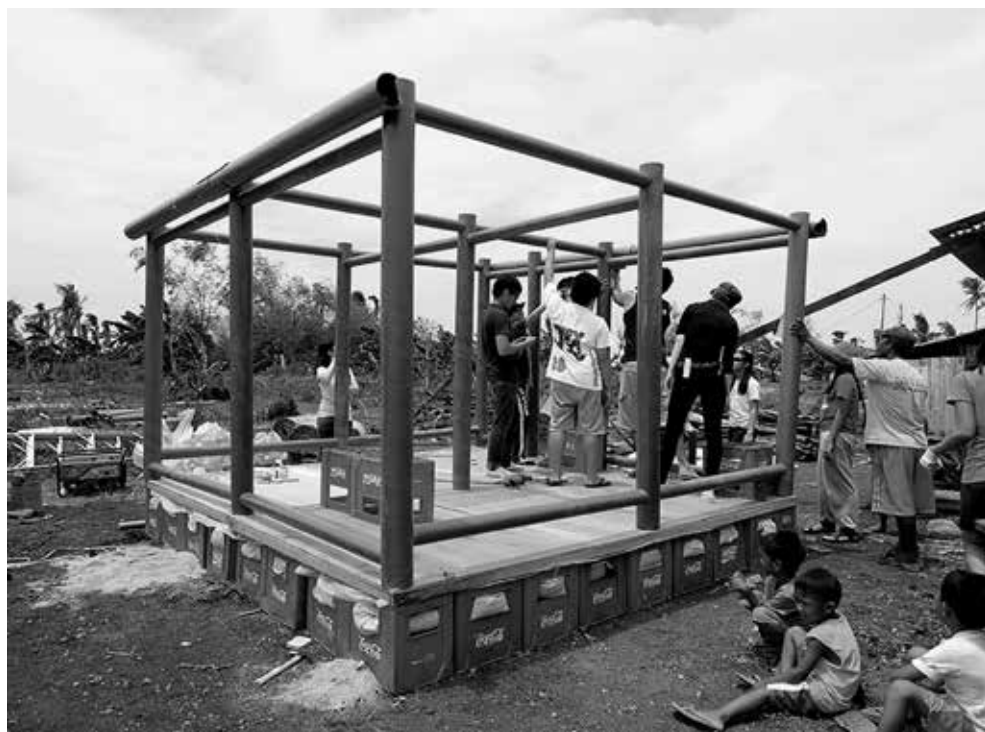
Ill. 5. Shigeru Ban, Paper Log Houses II, Cebu, Philippines, 2014. Temporary shelter made from cheap and generally accessible materials and construction waste. Ban combines such materials with local crafts, here with pleated bamboo mats and the nipa palm leaf roofs. Source: Jodidio P. Shigeru Ban. Complete works 1985–2015 , Taschen, Köln 2015.
