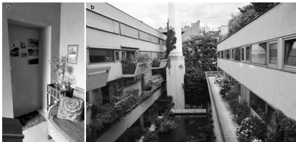
III. 4. BKK-2, Sargfabrik, Vienna, 1994–2000. Platform at one of the open staircases as an extension of a flat (a) and interior of the main courtyard, with the chimney of the former coffin factory as its dominant feature (b). Photo by the author.
