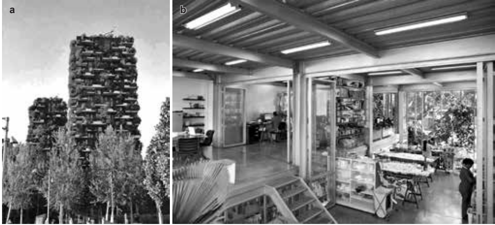
III. 5. a) Stefano Boeri, Bosco Verticale, Milan, 2007–2014. Present interpretation of a modernist tower – a facility in a park complying with principles of functionalism; here an enigmatic glass curtain wall has been replaced with a park with 800 trees. Photo by Hassan Bazazzadeh. Husos Arquitectos, Host and Nectar Garden Building, Cali, 2012; b) Venue of vocational activation of women and at the same time, a local centre of culture and a habitat of thousands of caterpillars, butterflies and birds, source: https://www.metalocus.es/en/news/bioclimaltical-prototype-accommodating-and-nectariferous-garden-building-husos (access: 26.09.2022).
