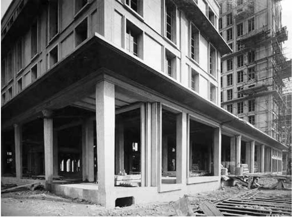
III. 2. Le Havre. Reconstruction of the port city between 1945 and 1964 – a reinforced concrete structure, based on repetitive structural modules, creating the modern character of the post-war centre, designed by August Perret and his team. Source: https://archimaps.tumblr.com/post/3944842368/reconstruction-of-le-havre-1945-64-france (access: 20.06.2022).
