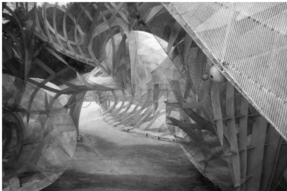
Ill. 5. Son-O-House Sound Pavilion in Eekersrijt, the Netherlands, view of interior – the space of sound imagination, photo by E. Cisek.
