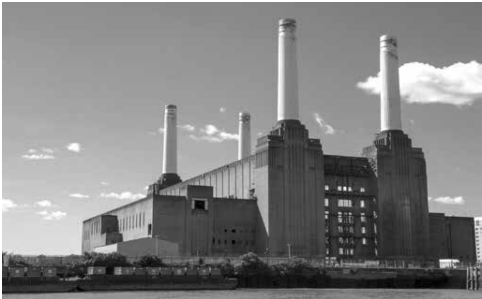
Ill. 1. Battersea Power Station, G.G. Scott, London 1939, 1953–1955, photo: Alberto Pascual.
