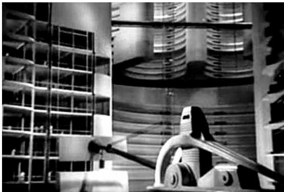
Ill. 3. Installation of buildings from prefabricated concrete elements in the film “Things to come” 25 .
