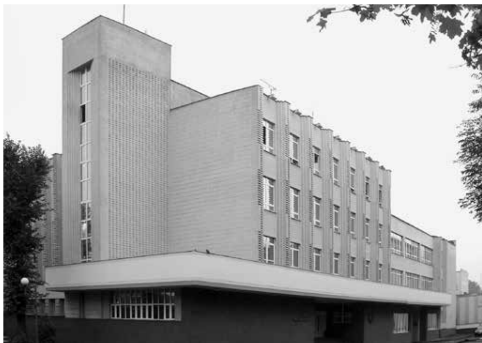
III. 4. Railwaymen's Palace in Lviv. Arch. R. Miller, 1938. Source: https://top-tour.lviv.ua/ru/ukrayinska-lviv-na-kistkah-abo-znikli-tsvintari-lvova/ (access: 5.10.2022).
