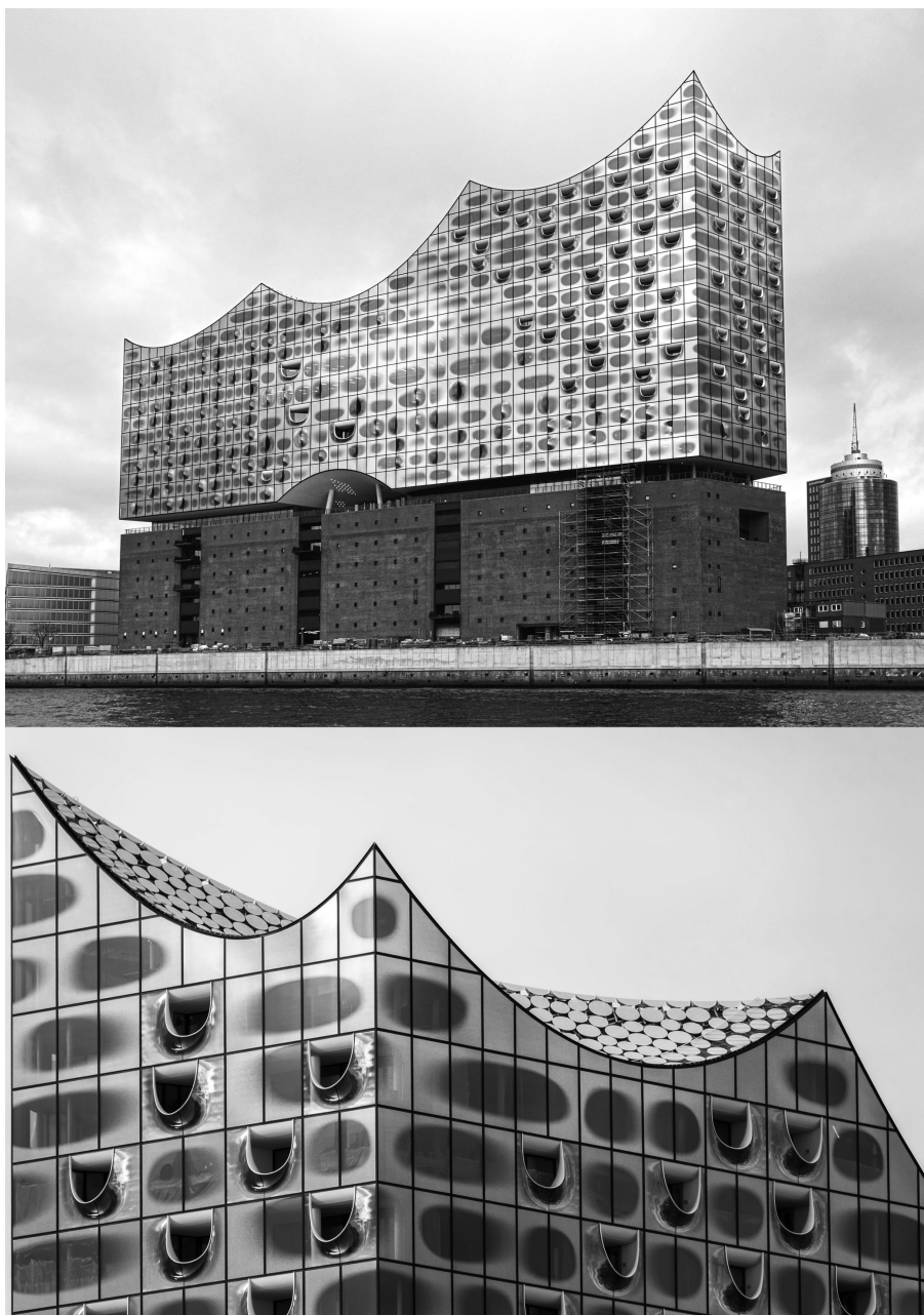
III. 1. Top picture – view of the facade of the Hamburg Philharmonic from the side of the Elbe River. Source: https://www.pikist.com/free-photo-sizls/download/pl (access: 20.06.2021); below – close-up view of the glass facade and the curved roof. Source: https://www.pikist.com/free-photo-sizls/download/pl (access: 20.06.2021).
