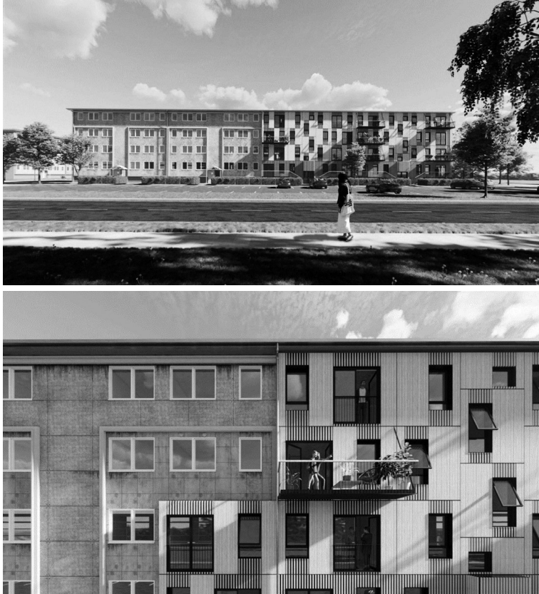
Ill. 7–8. REBUS – a prefabricated solution for existing building facades, designer H. Larsen, source: https://henninglarsen.com/research/insights/2020/09-to-improve-social-housing-our-approach-is-keeping-the-old-and-making-it-better/ (access: 24.06.2021).
