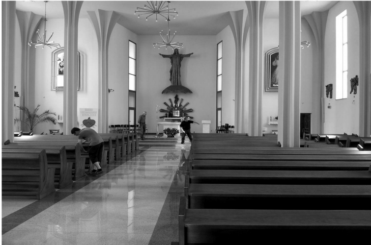
Ill. 3. Mushroom-shaped concrete pillars supporting a flat ceiling in the church on Gotyk estate in Krakow, intended to expose the concrete, unfortunately finished with the same paint as the walls, designed by B. Podhalański.
