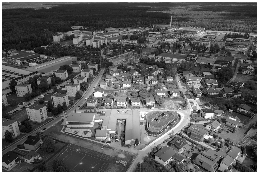
III. 3. M. Konopnicka Kindergarten, TOPROJEKT, Żory, Poland – the bird's eye view of school and kindergarten complex with oval kindergarten building. Source: http://www.topprojekt.com/projekty/przedszkole-zory-kleszczowka/ (access: 21.06.2021).
