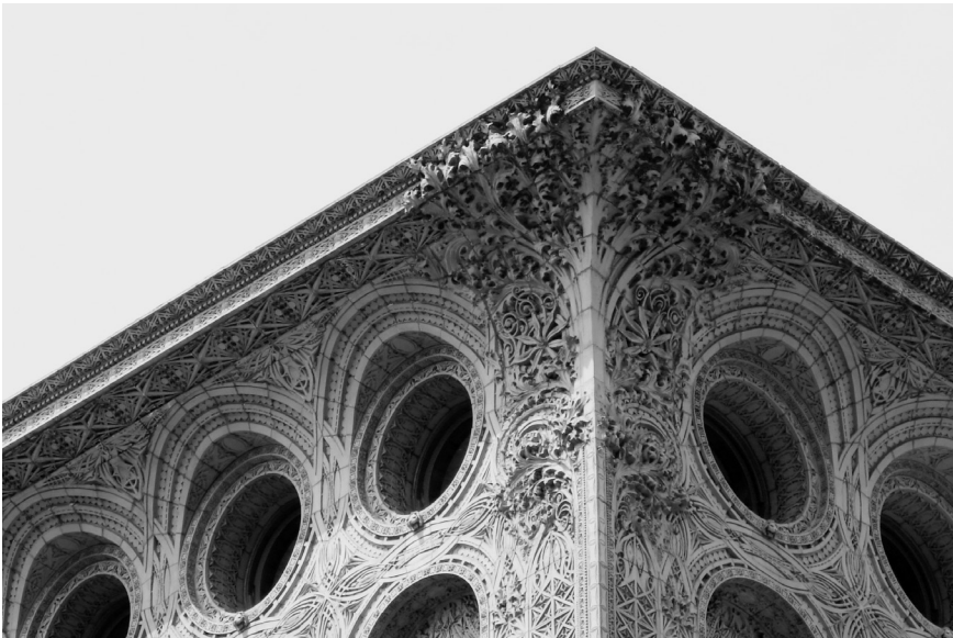
III. 4. Buffalo NY (USA). Prudential Guaranty Building, 1895-1896. The crowning cornice. (Author: Louis H. Sullivan & Dankmar Adler). The example which confirms that the author of the statement “form follows function” perceived both functionalism and decoration in architecture differently than the modernists. Source: Michał Domińczak ©.
