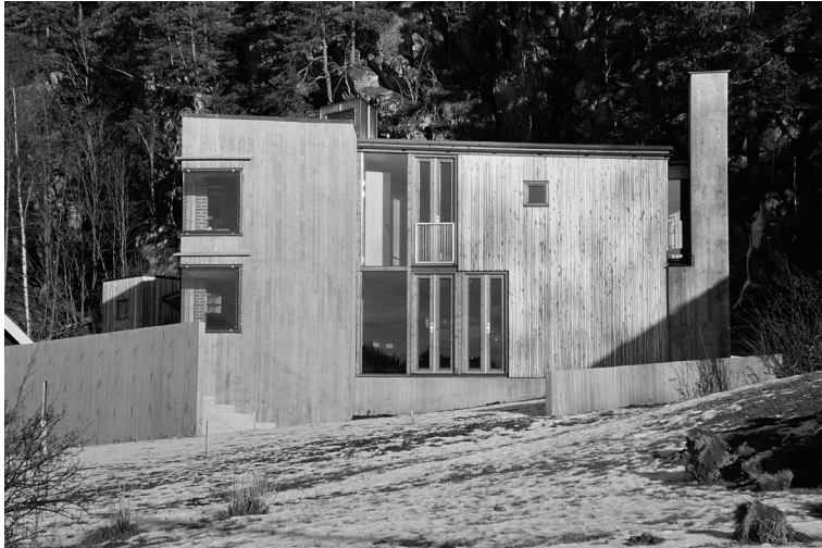
Ill. 5. Holme Studio in Hurum by Sverre Fehn, Norway, 1996, source: https://www.arkitektur-n.no/prosjekter/atelier-holme-hurum?cat=2710 (access: 10.06.2021).
