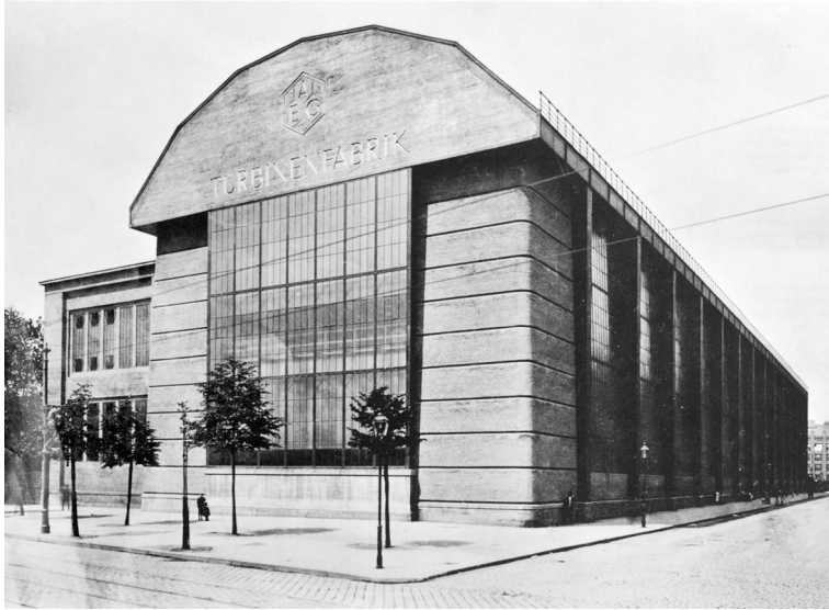
III. 1. Peter Behrens, Turbinenfabrik, Mantagehalle, Berlin 1909, front façade (from Fritz Hoeber, Peter Behrens , München 1913).
