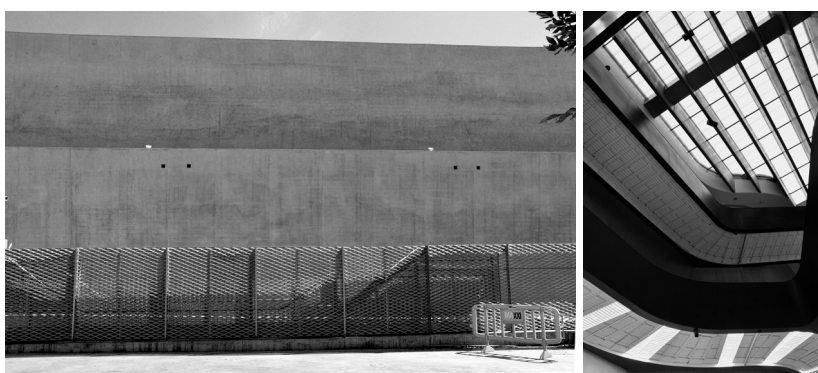
Ill. 4. Maxxi Museum. Massive fence and façade facing Via Luigi Poletti – the opposite of the building, which, according to Hadid, is organised and navigated on the basis of directional drifts and the distribution of densities rather than key points . This is indicative of the character of the Centre as a whole: porous, immersive, a field space (Noever P. (ed.), Zaha Hadid. Architektur/Architecture , Hatje Cantz, Ostfildern 2003). Photos by the author.
