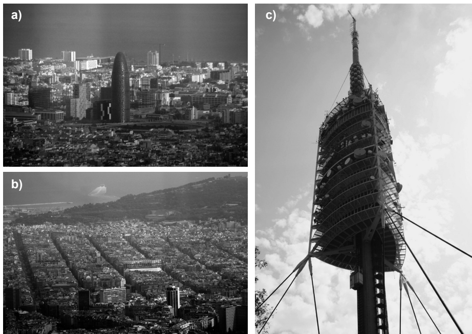
III. 1. Barcelona, a) panorama of the city seen from the radio and television tower, b) view on Torre Agbar, Jean Nouvel, Fermín Vázquez Huarte-Mendicoa, c) Torre de Collserola, Norman Foster, Barcelona. Photos: K. Słuchocka.
