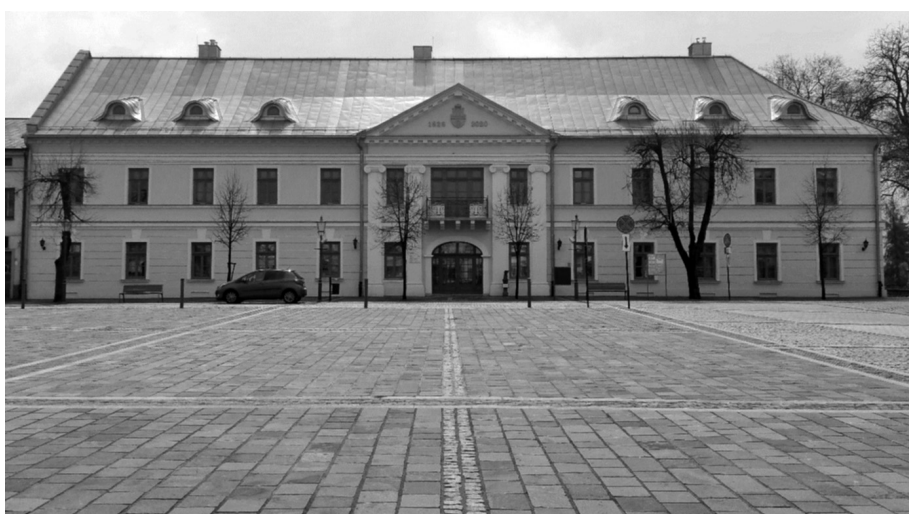
III. 6. Change in the use of the object as a result of social, economic and technological conditions. Former Starosty Building in Olkusz – today a Muzeum; above – before, below – after revitalisation. Photo by G. Nawrot.
