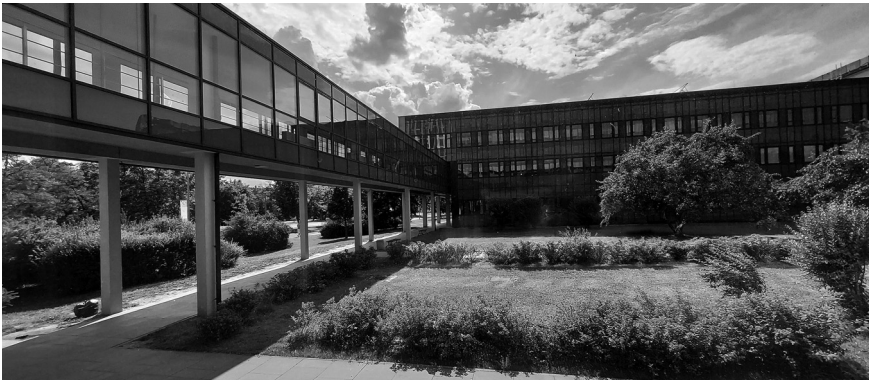
Ill. 3. Faculty of Mechanical Engineering building – internal courtyard, photo: author
